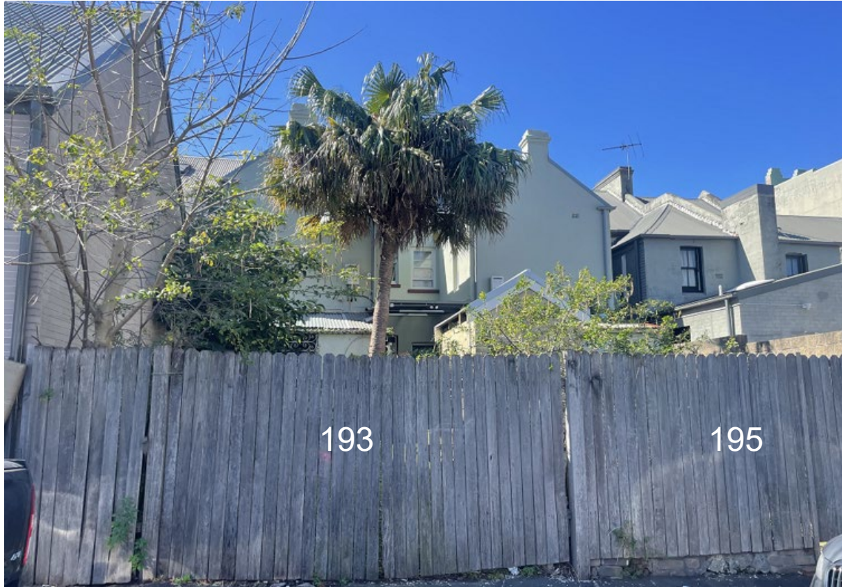
rear of site - Little Mount Street
