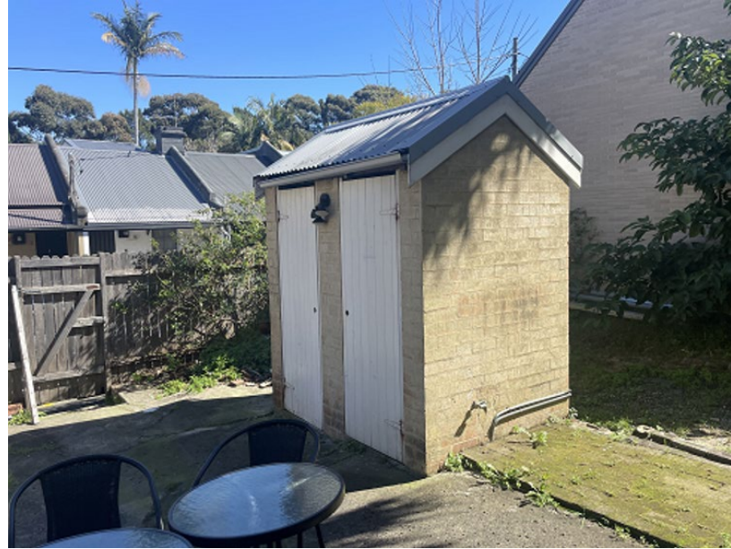
outbuilding to be demolished and boundary adjusted
