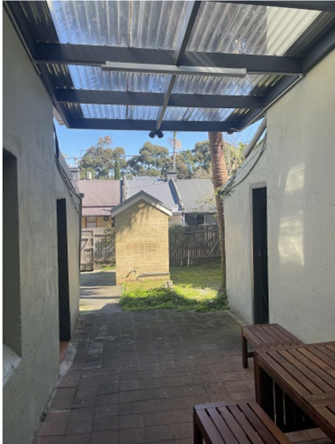
ground floor rear wings with shared communal open space to rear
